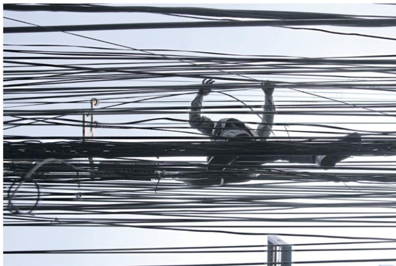
An electrician walks above tangled power, cable TV and telephone lines during maintenance work on Ngam Wong Wan Road. WICHAN CHAROENKIATPAKUL
