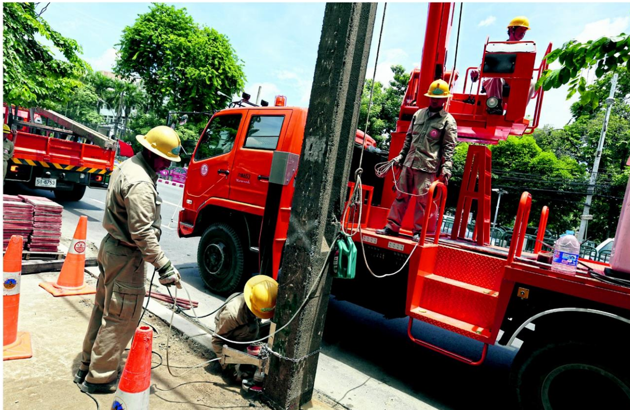
Staff of the Metropolitan Electricity Authority of Thailand remove power poles on Ratchawithi Road, in line with the MoU to relocate all overhead power lines and cables underground. THANAPHON ONGARTTRAKUL
