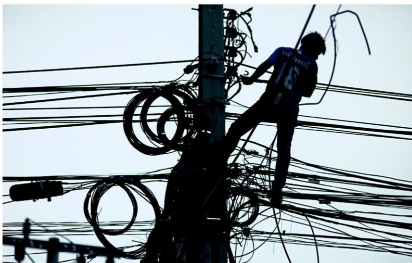
A technician installs telephone cables at the Uruphong intersection in Bangkok. The NBTC may impose stricter measures on the installation of mobile towers. PATIPAT JANTHONG
