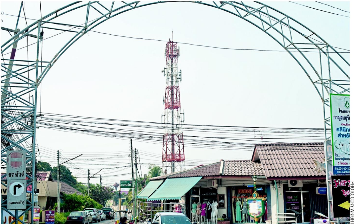
WIRES CROSSED: The increasing number of towers in populated areas like this one in Kanchanaburi have some concerned about adverse health effects.
