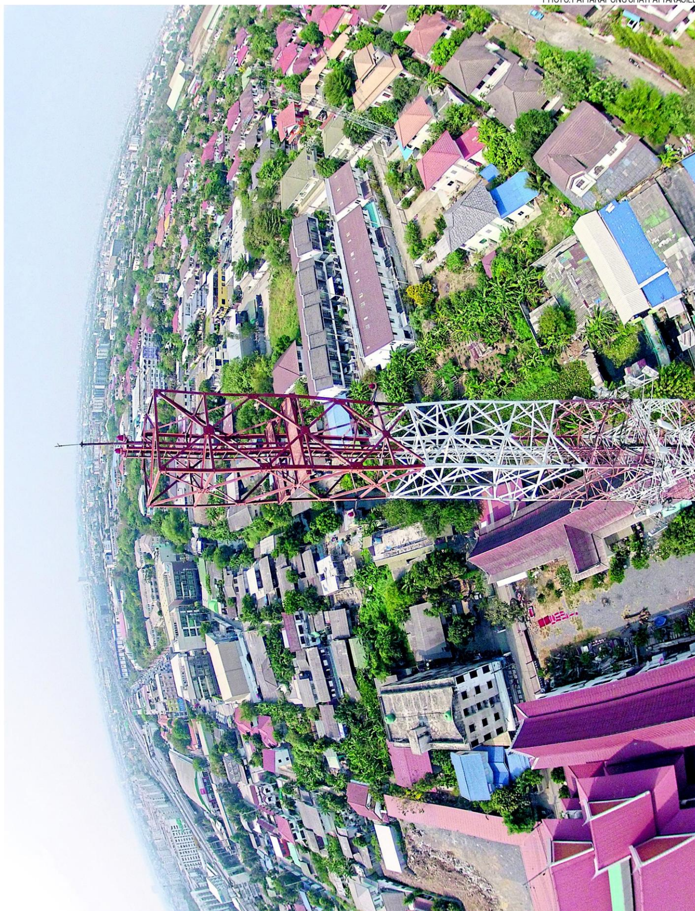
FREQUENT COMPLAINTS: Chaiyapruke Ramintra estate has seven towers and one base station nearby, leaving residents worried about exposure to radiation. Thailand has more than 60,000 phone towers.
