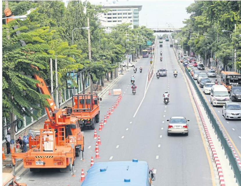
The Metropolitan Electricity Authority started putting power cables underground at Ratchawithi Road in September 2016. TANAPHON ONGARTTRAKUL
