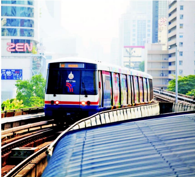
Early next month TOT will start the trial of non-commercial wireless broadband service on its 2.3GHz band along selected sections of the Skytrain routes above Phaholyothin Road, Sukumvit Road and in Ratchaburi province.
