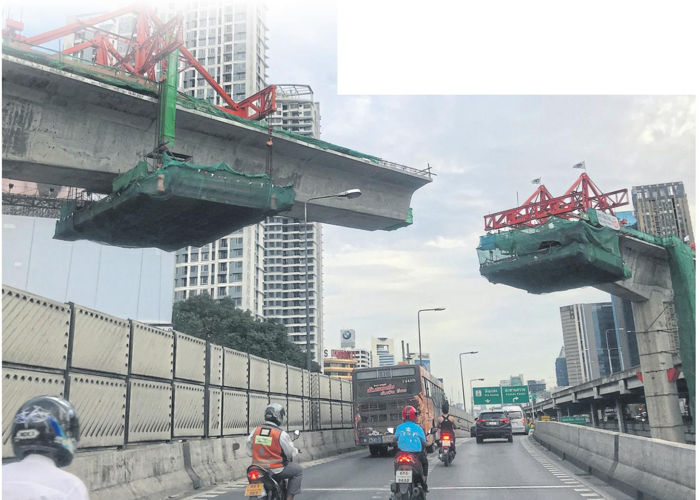
Construction of the Light Green Line extension (Mor Chit-Saphan Mai-Khu Khot) is under way, with service to begin in 2020. PATTANAPONG HIRUNARD
