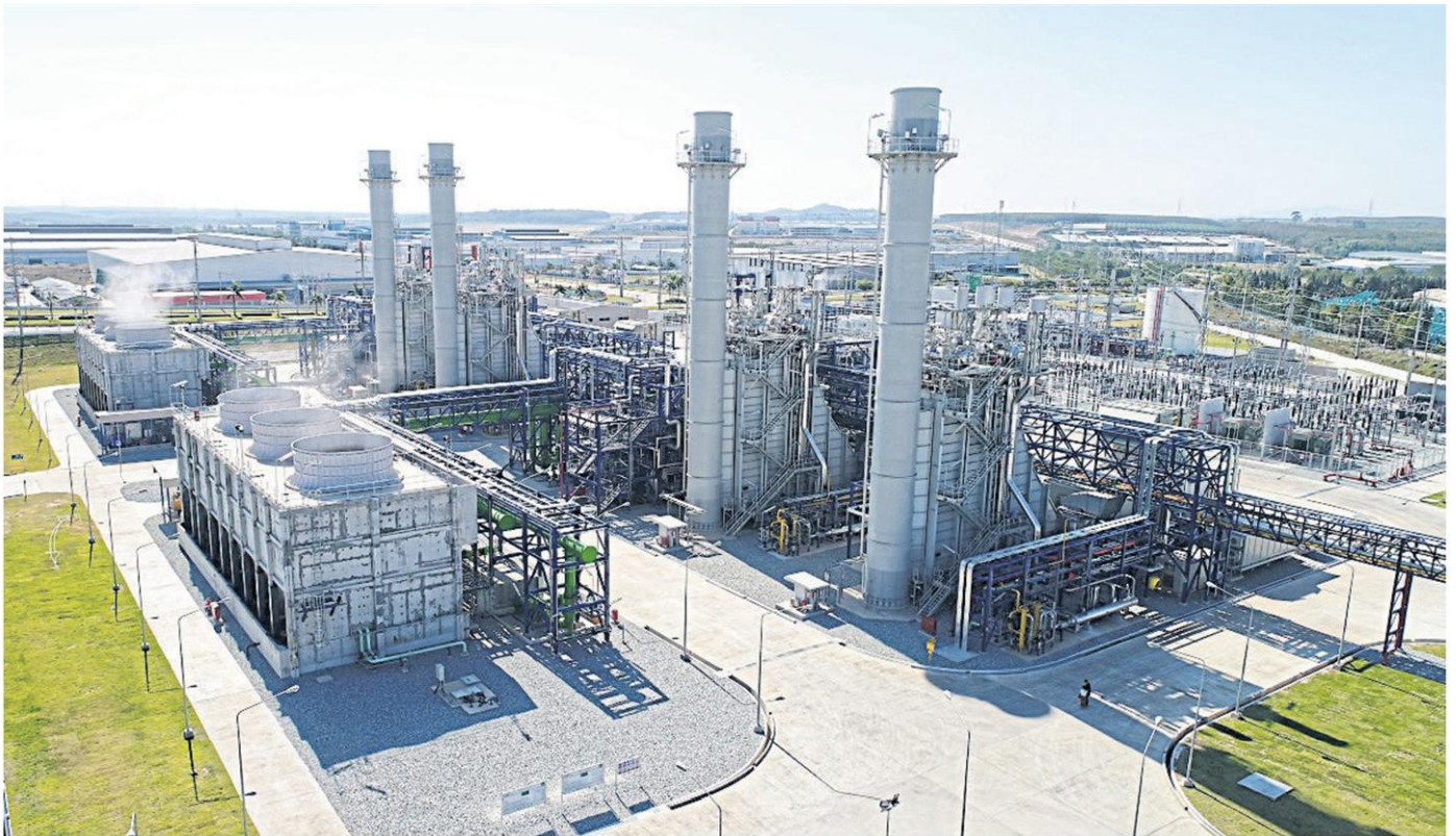
Gulf Energy Development's power plant at Hemaraj Eastern Seaboard Industrial Estate.
