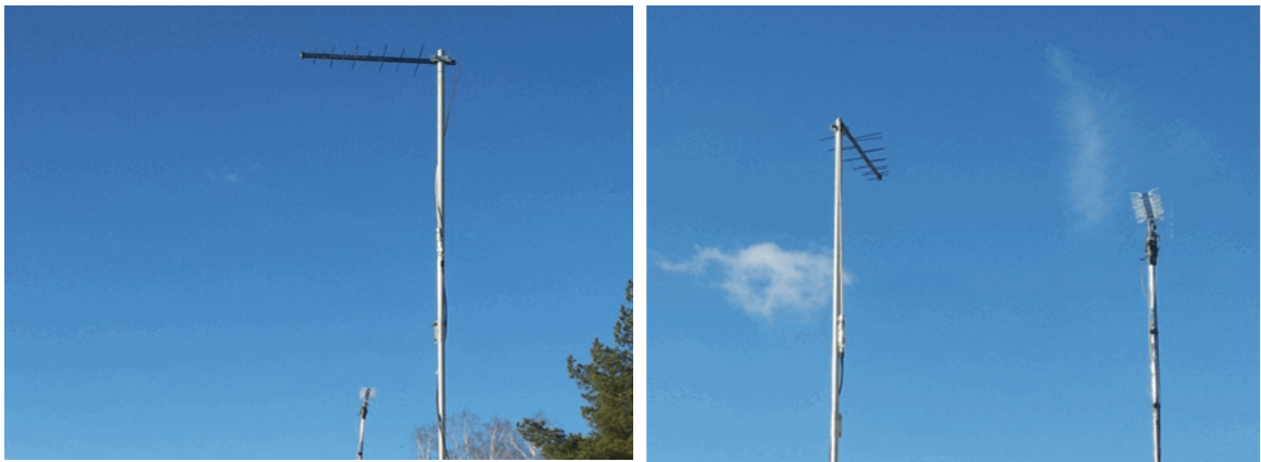
FIGURES 46 AND 47 Positions of TV broadcasting receive antenna and fixed wireless broadband access system transmit antenna
